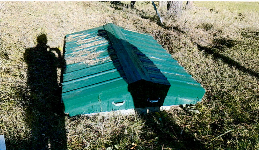
Palmer Rd well pit cover
