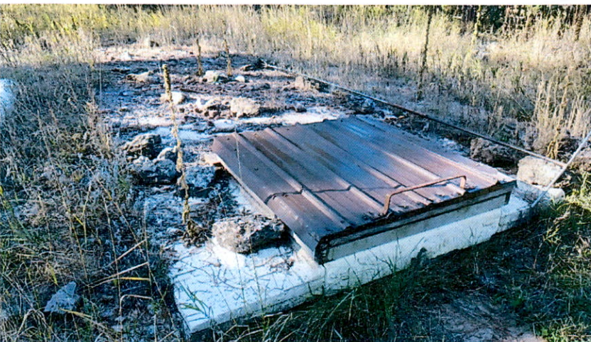
Palmer Rd. storage reservoir
