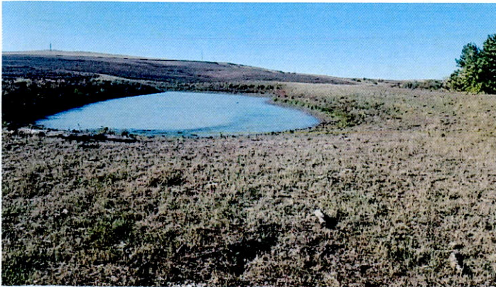
Diversion dam and pool
