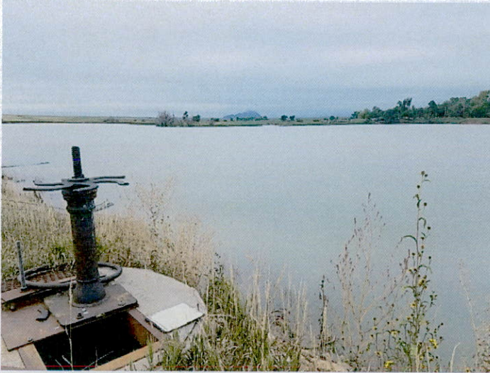
pool with riser and slide gate handwheel
