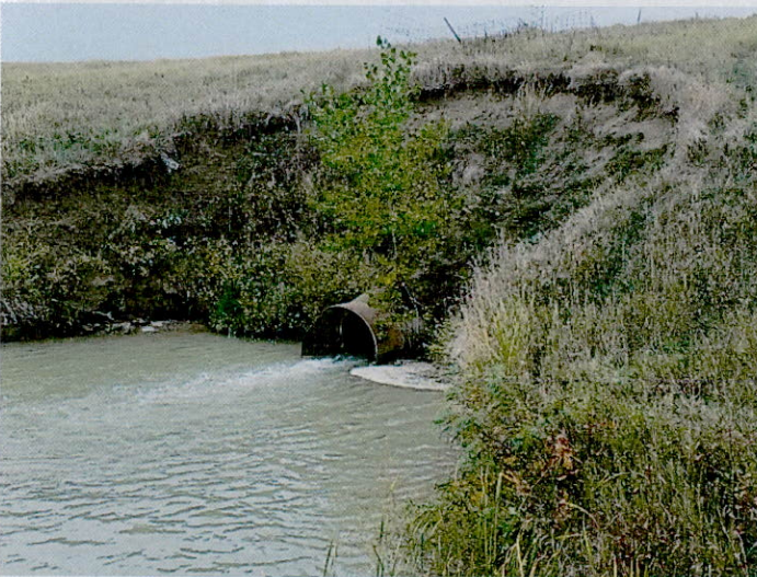
spillway outlet
