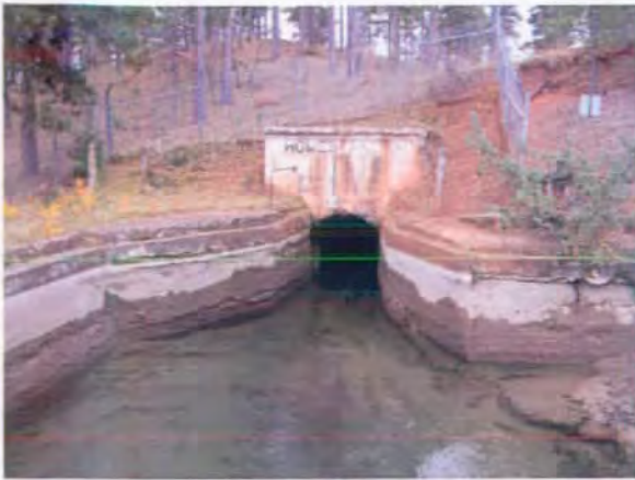
Forebay Dam. Entrance Portal
