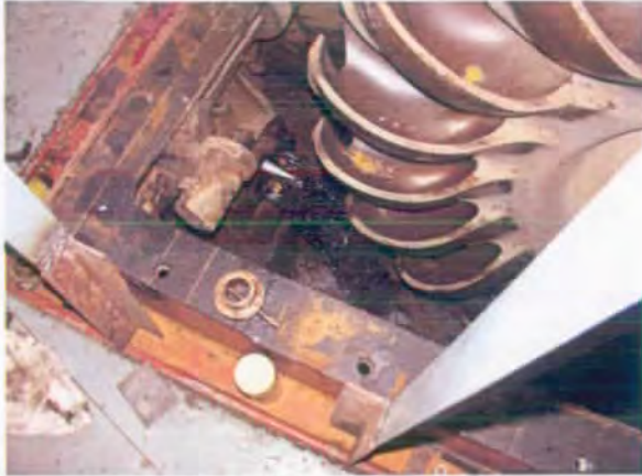
Pelton Wheel and Nozzle
