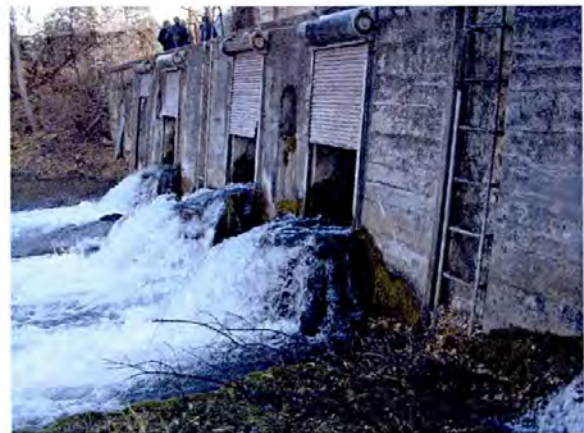
Powerhouse. Water Return
