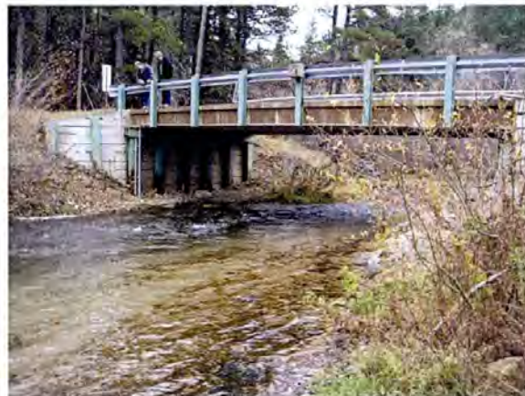
USGS Maurice Gage. Sensor Location Site
