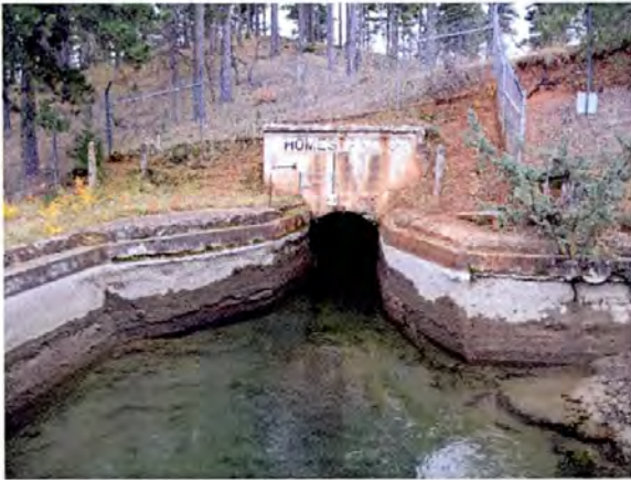
Forebay Dam. Entrance Portal
