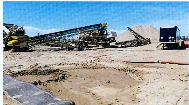
Gravel washing operation
