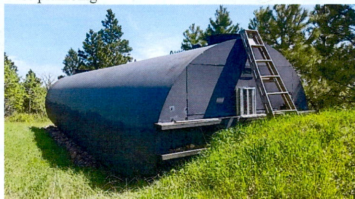
44,000 above ground steel storage tank
