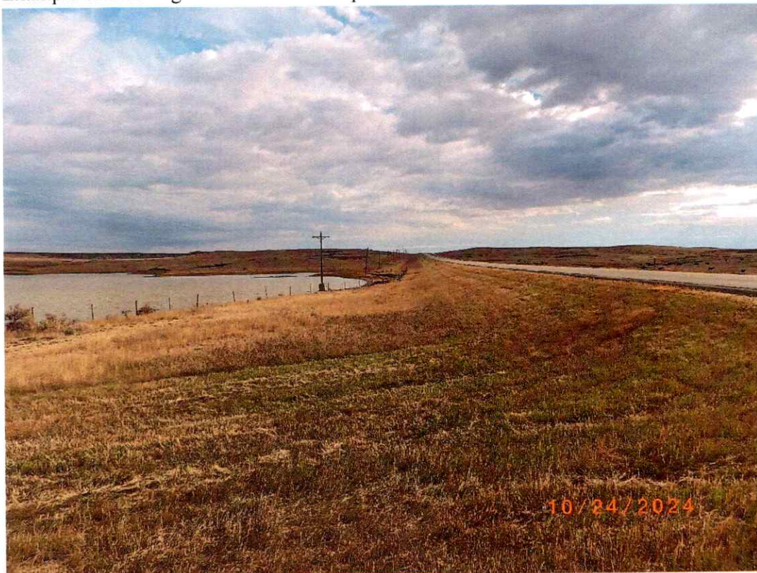
Dam overview picture. Note cattle in the downstream area.
