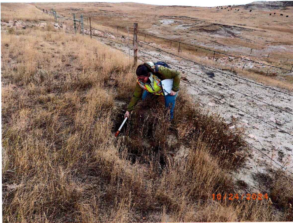
Picture shows approximat location of downstream sinkhole. Note lack of grass cover in grazed area of the slope.
