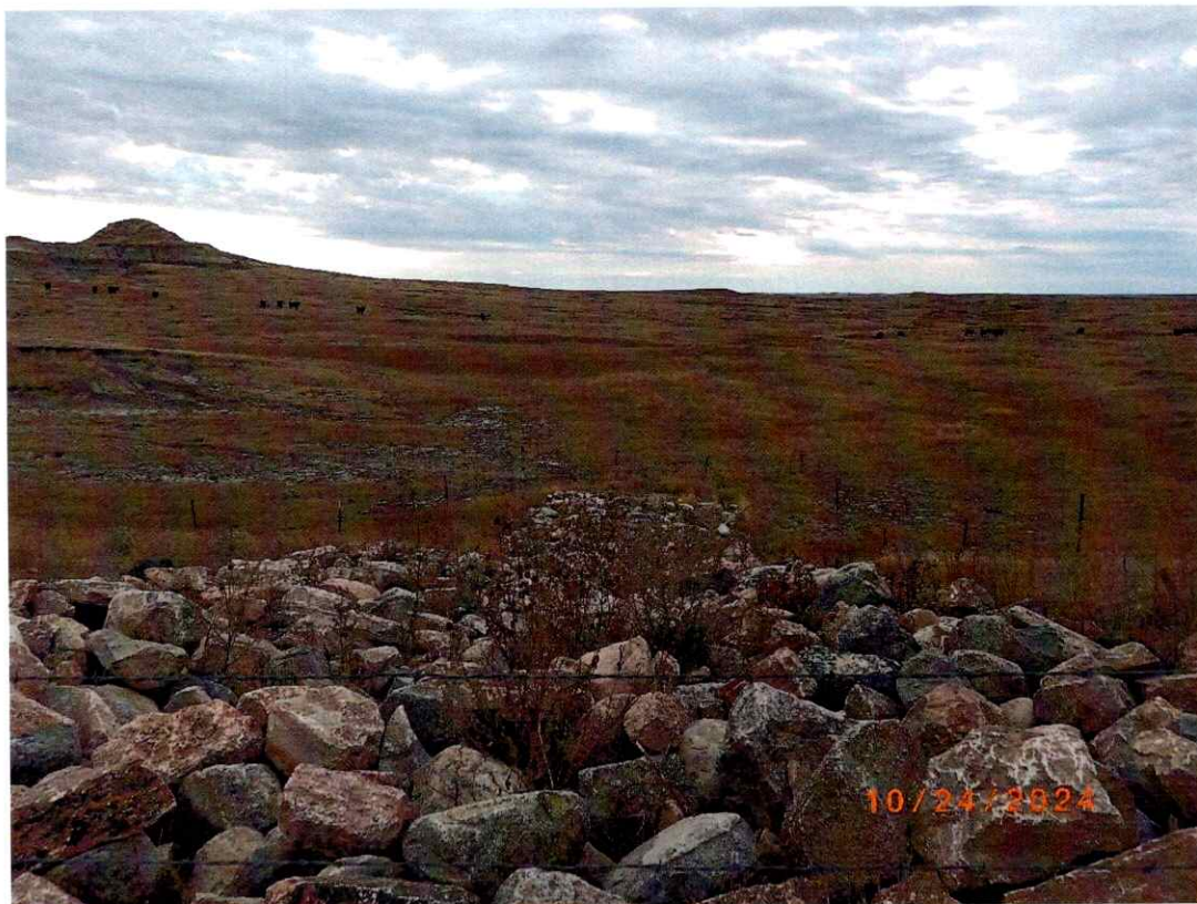
Ripraped channel below conduit outlet.
