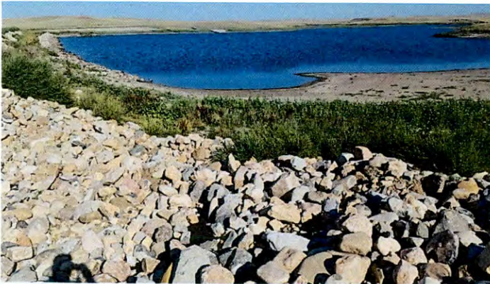
Inlet to spillway, pool, and riprap along dam front face
