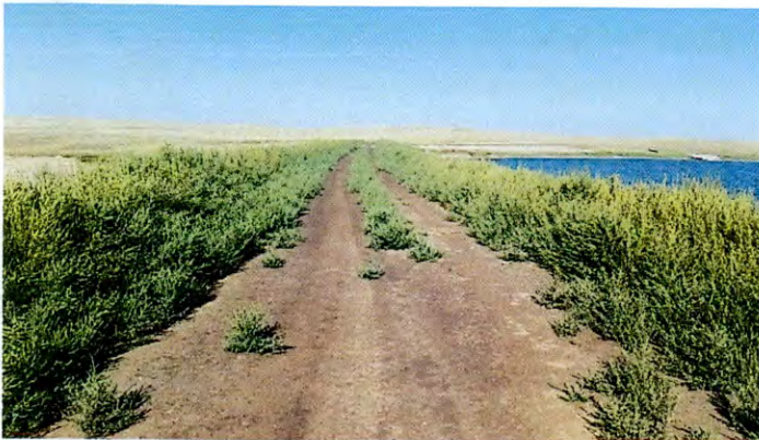
Crest of dam viewed from east end.
