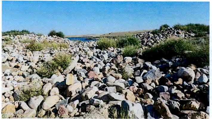
Outlet of spillway looking towards inlet and pool
