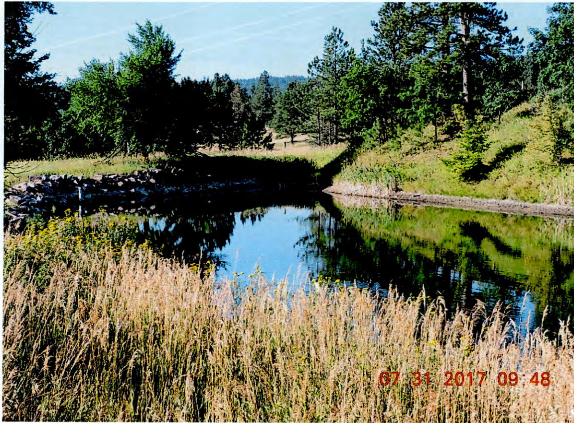
Pond #2 – facing downstream in a southwest direction. Note the line indicating previous water surface elevation.
