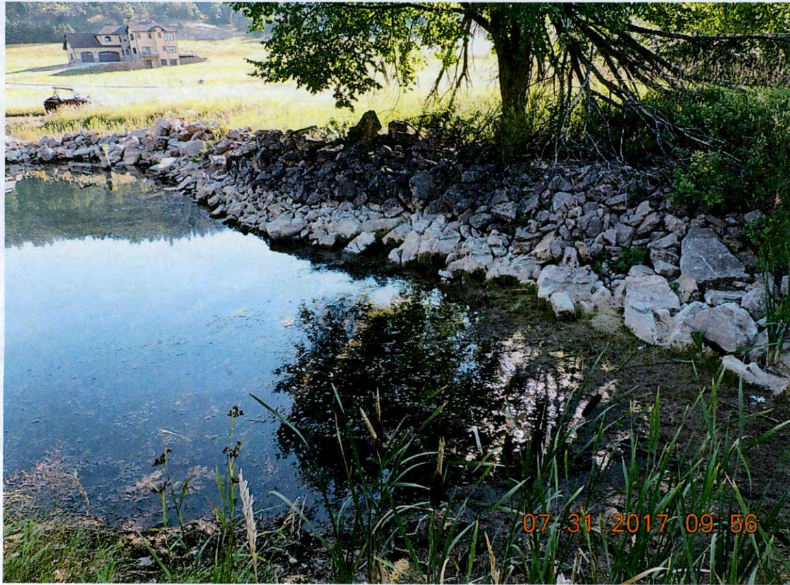
Pond #2 – facing east looking across the face of the dam. Note the current water surface and evidence of previous water level.
