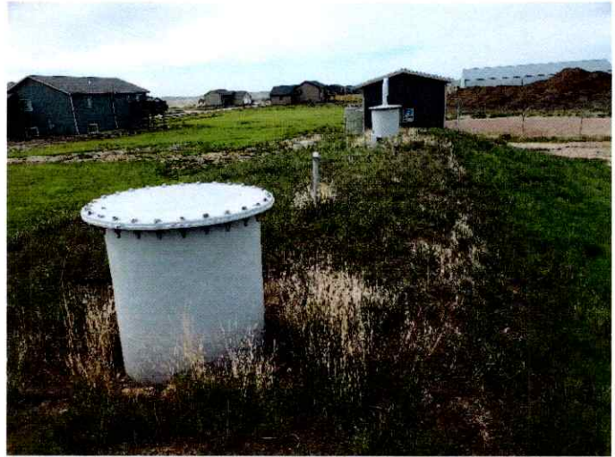
Fiberglass storage access manholes with pump house in background
