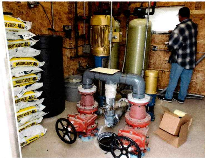
Pump house appurtenances
