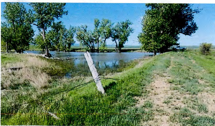
East end of fill (view to west) with spillway at left
