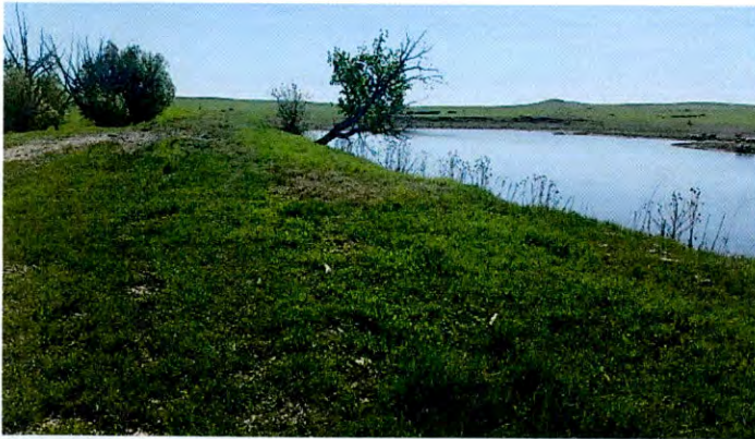
Top of dam and pool
