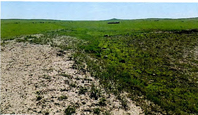
Looking to east at spillway and diversion
