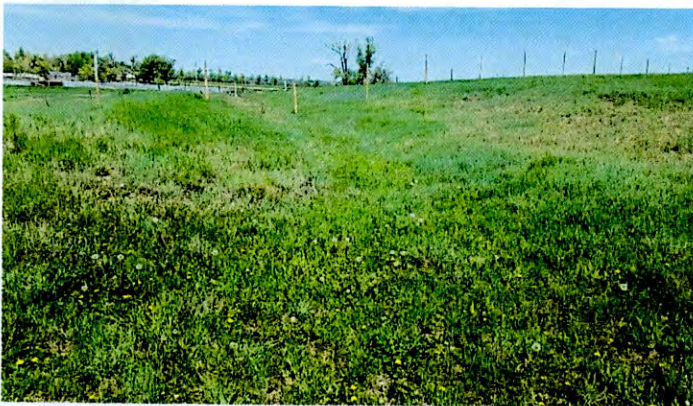
Earth spillway, looking to northwest
