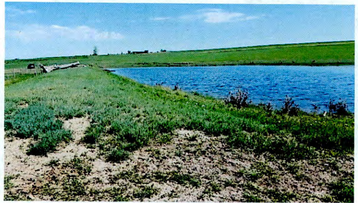
Embankment and pool, looking to north
