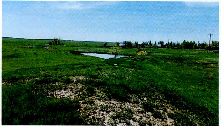
Embankment and earth spillway (center left)
