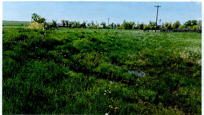
Backslope of dam and twin 8" PE drain tubes
