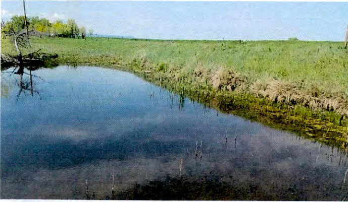
Front Slope of embankment, invert of 8" tubes @ waterline
