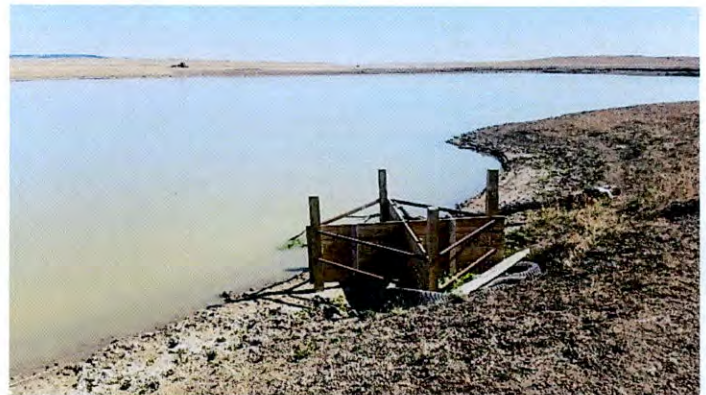
Primary Spillway inlet and pool
