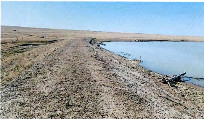
Crest of dam
