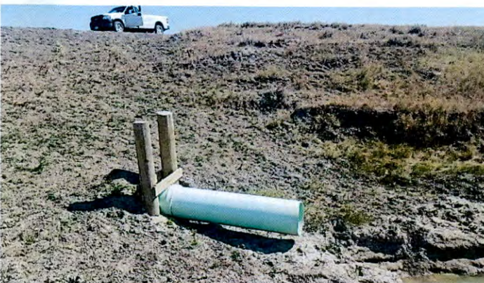
18" PVC spillway outlet
