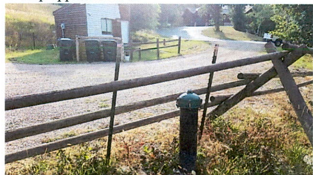
2015 well and pump house
