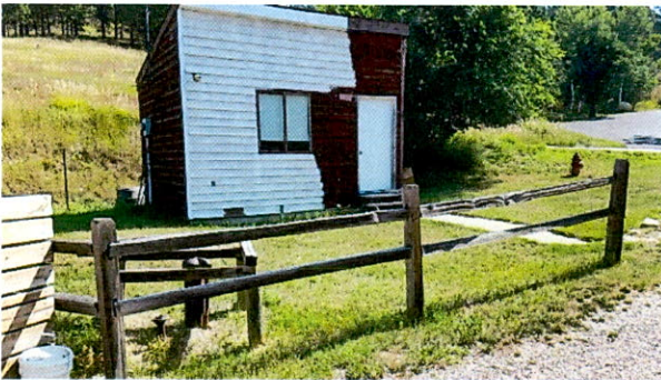
Stand-by Well and pump house
