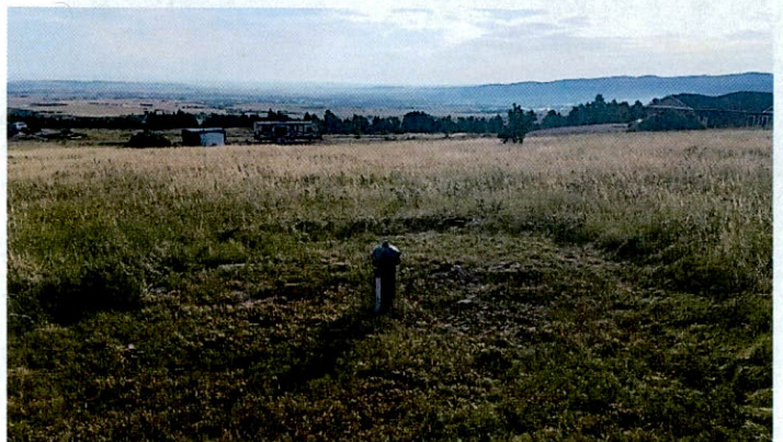
2008 well for upper system (standby)
