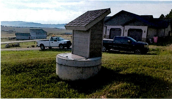
South well pit (1972) and shelter for chlorinator
