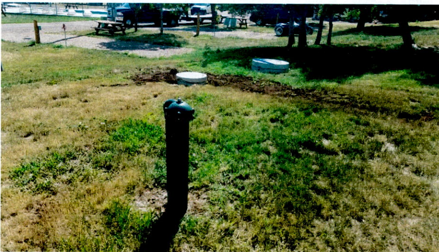
Well head with cistern and booster pit in background
