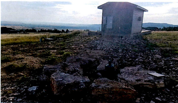
2015 well, pump house and 46,000 gallon storage
