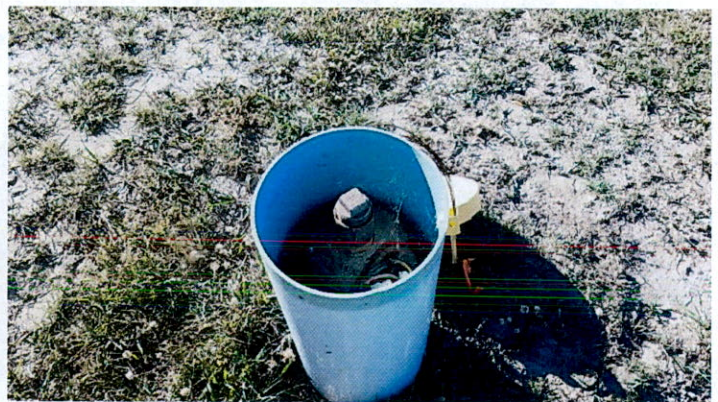
well cap inside protective enclosure
