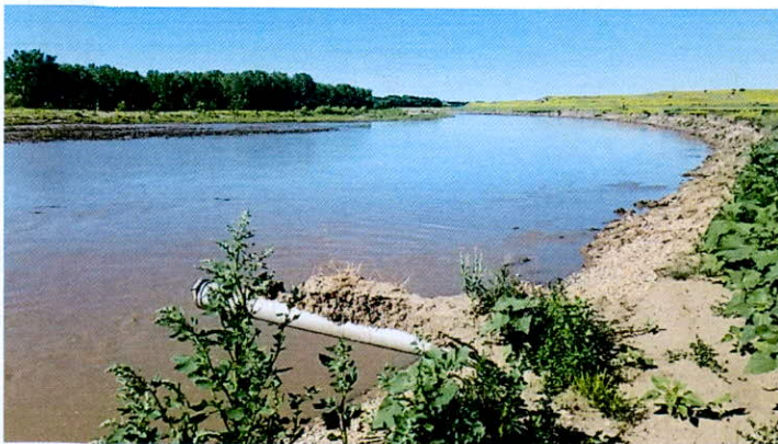
Belle Fourche River diversion location 6/27/19
