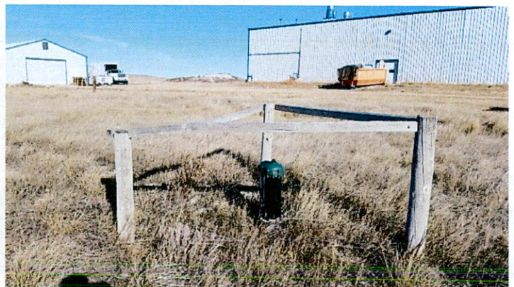
well with garage to upper left and plant to upper right
