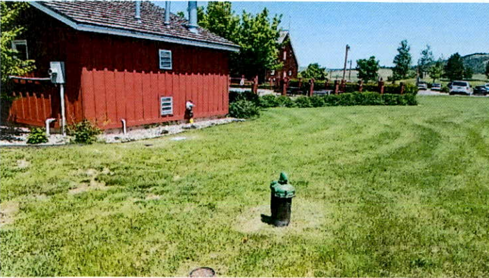
Well with pump house @ upper left
