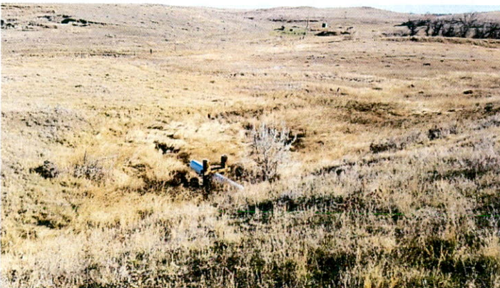
PVC principal spillway outlet
