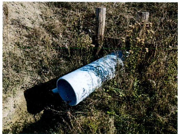
PVC spillway outlet
