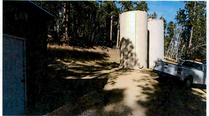
Twin 25,000 gal. storage with well house in foreground
