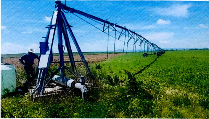
Pivot and manifold with Air/Vac valve
