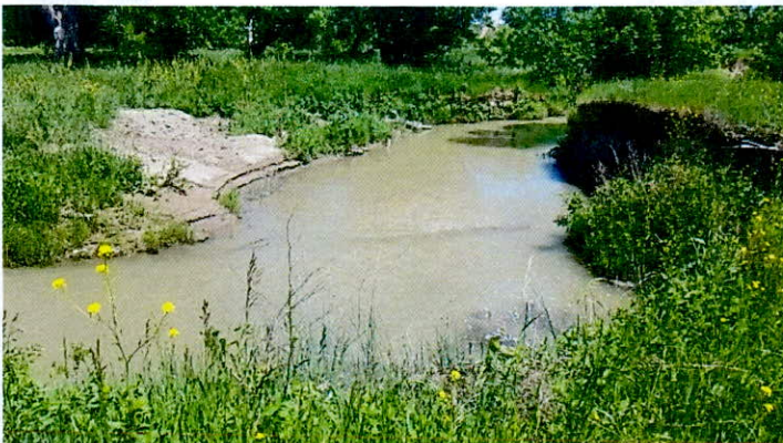
Nine Mile Creek diversion 6/19/2019
