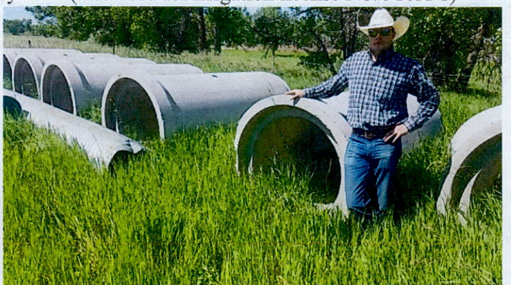
36" concrete pipe used for twin diversion intakes
