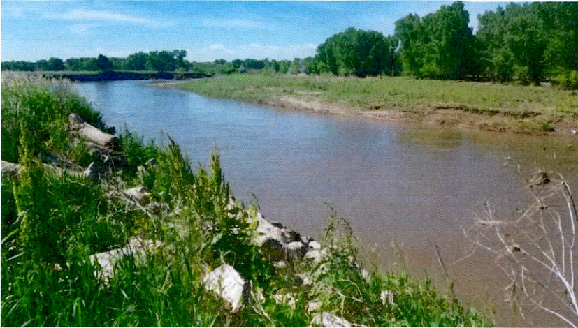
Belle Fourche River diversion location. Water is diverted to the pumping gallery through twin 36" concrete pipes approximately 430' long.
