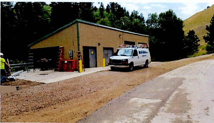
Yates Water Treatment Plant
