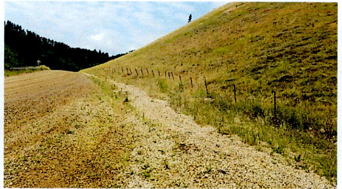
Looking west along Kirk Road and toe of waste rock
