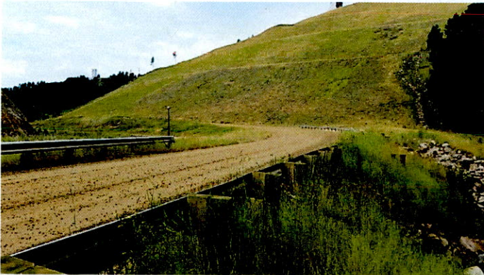
Looking west along Kirk Road and toe of Yates Waste Rock site. The 6" HDPE collection pipe is located along slope the the right side of the road at the base of the waste rock slope and crosses the road in the foreground.
