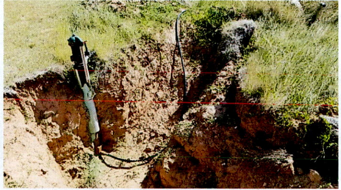
Temporary pipe connection to distribution
