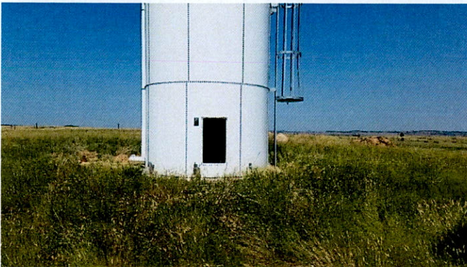
Storage tank with access door removed
