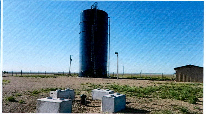
Well, storage and pump house
