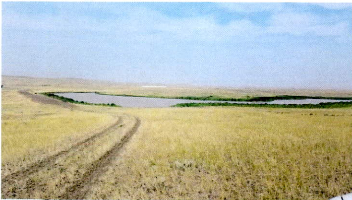
Pool and embankment
