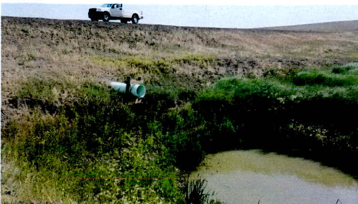
Principal Spillway outlet
