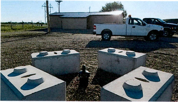
Well and pump house
