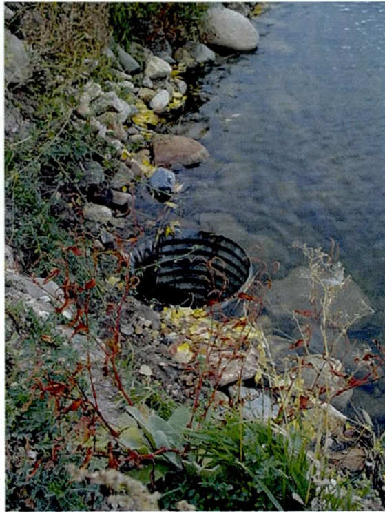
drop inlet structure estimated flow of 80 -100 gpm on October 21, 2005
