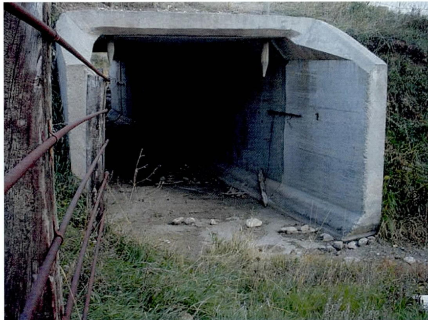
Picture of box culvert through road approximately 440 yards downstream of dam
