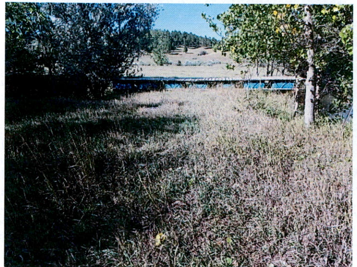
crest of embankment looking southwest
