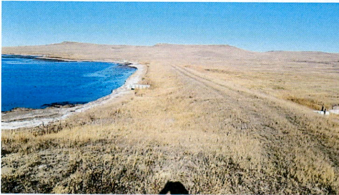
embankment, pool and outlet
