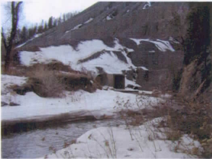
Photo 12. Upstream view of culvert outlet and toe of waste rock pile in the proposed channel relocation project site.
