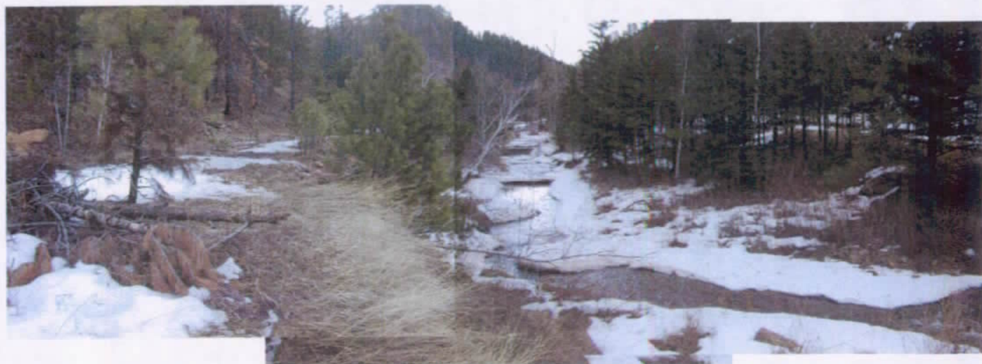
Photo 6. Downstream view of Whitewood Creek channel to be relocated. Photo taken immediately downstream from trail bridge.
