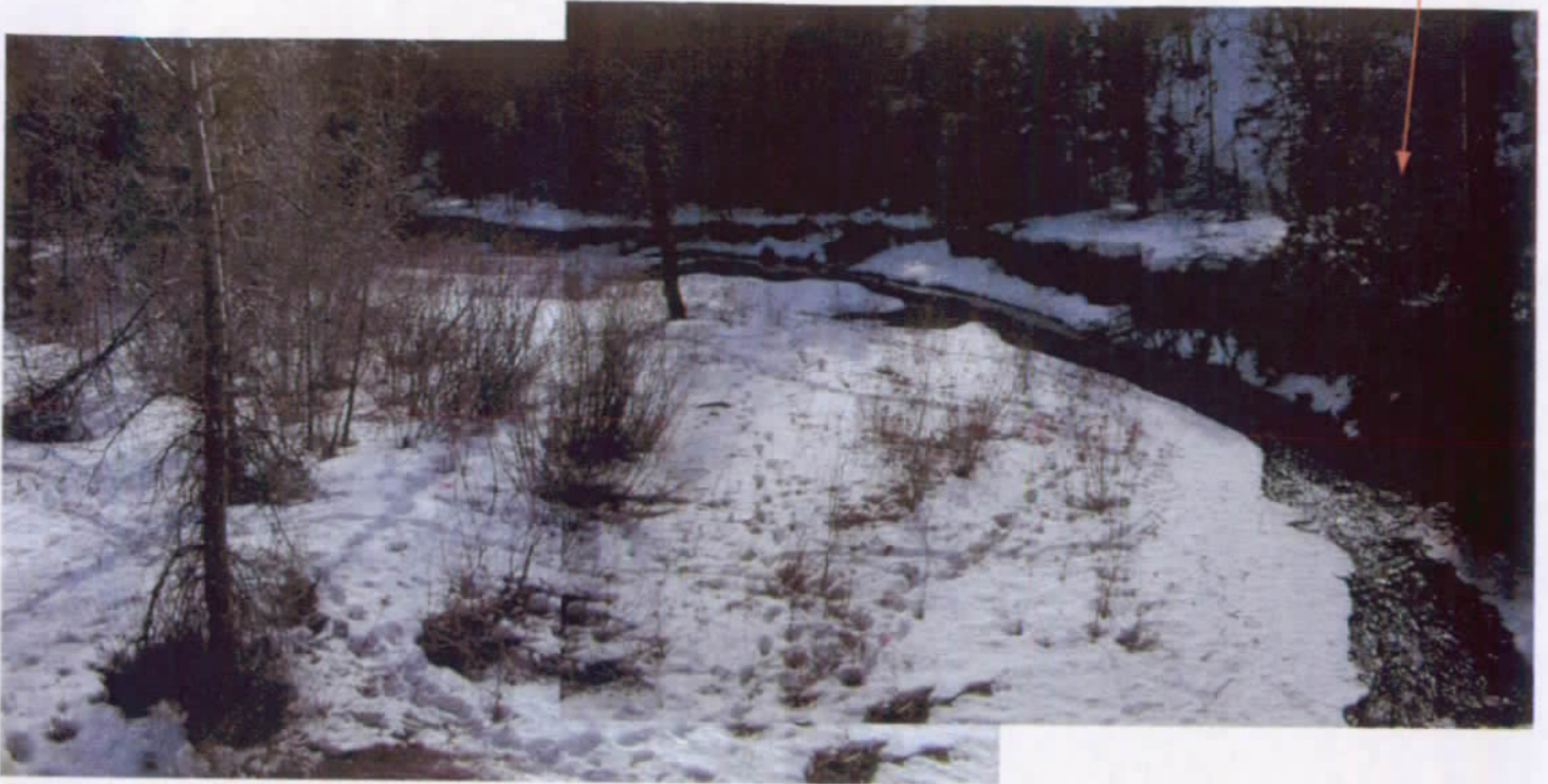
Photo 15. Downstream view of Whitewood Creek from foot bridge. Arrow indicates the connection point of the proposed relocated channel. Cutbanks on the far bank are approximately 8 feet above the water surface. Willows dominate the surface of bank in the foreground.
