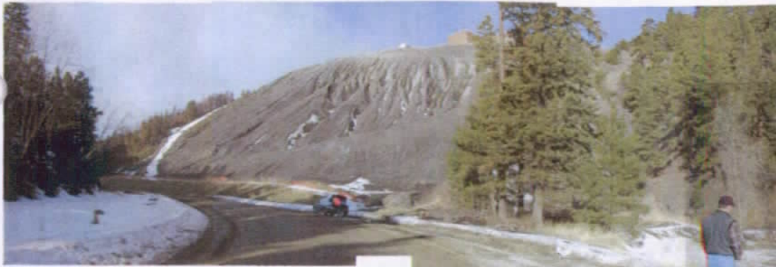
Photo 11. View of proposed channel relocation project area downstream from culvert outlets. Waste rock pile is in view. Arrows indicate location of the entrenched channel not visible from this view.
