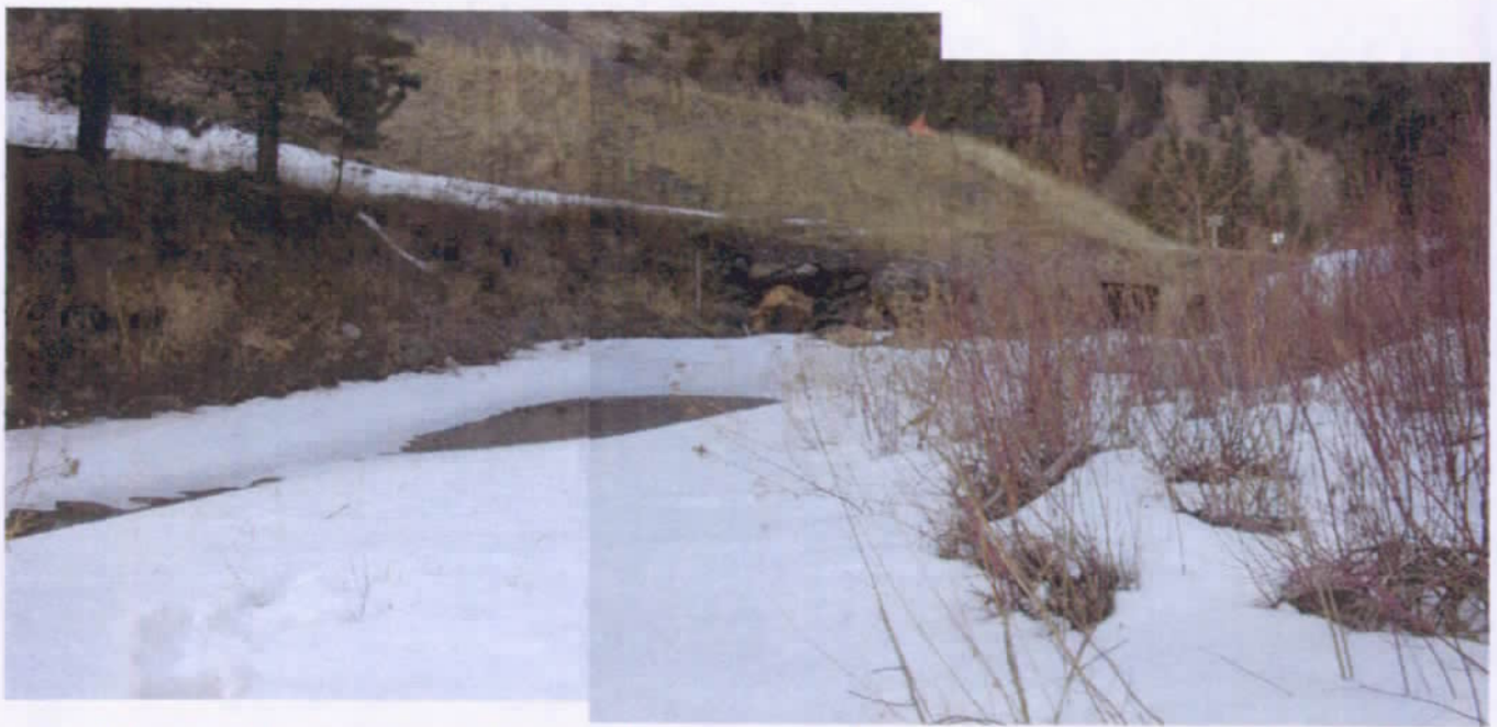
Photo 10. View of culvert inlet at the toe of waste rock pile. Note steep cut on the left bank. Redosier dogwood dominates the right bank in the foreground.
