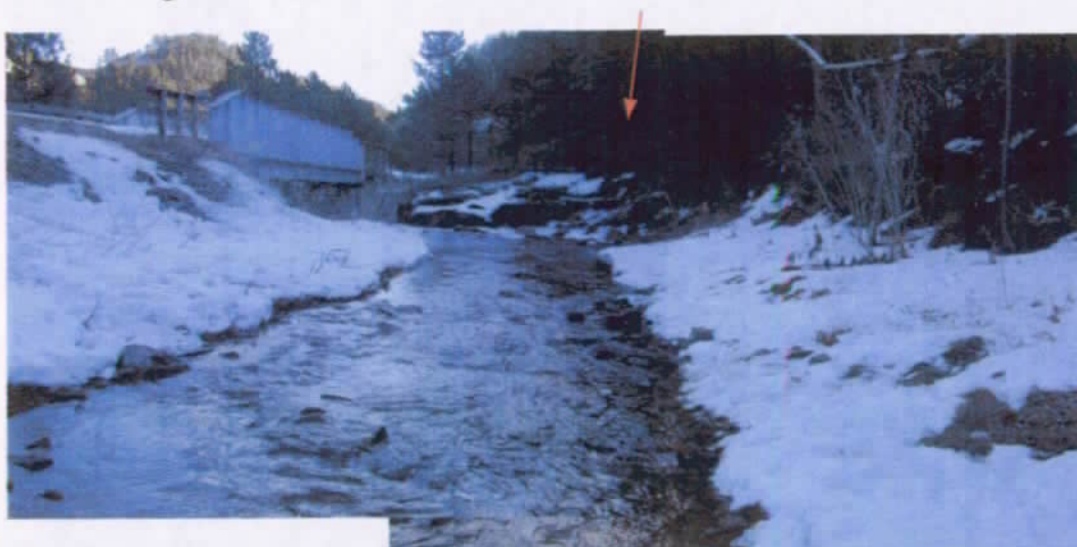
Photo 5. Downstream view from WC-T3. Arrow indicates the upstream begin point for the proposed channel relocation. Existing trail bridge is in view.
