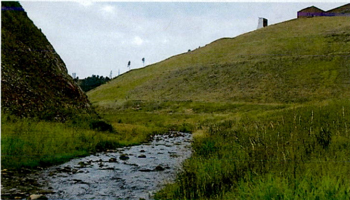
Looking upstream from lower end of constructed channel
