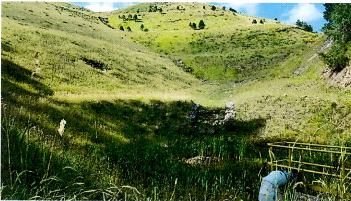
Bobtail drainage and surface water collection pond
