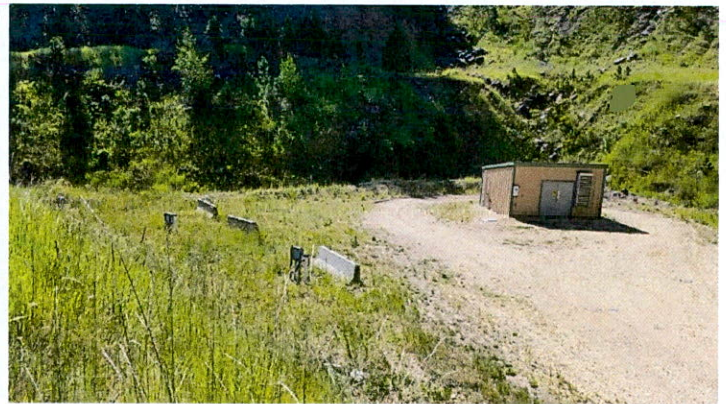
East Ravine collection wells (3)
