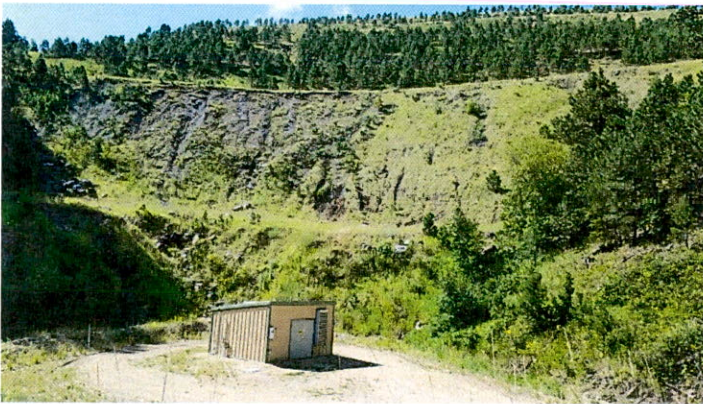
East Ravine drainage and pump site
