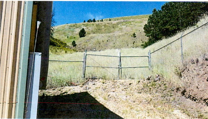
Sawpit Gulch drainage and pump site
