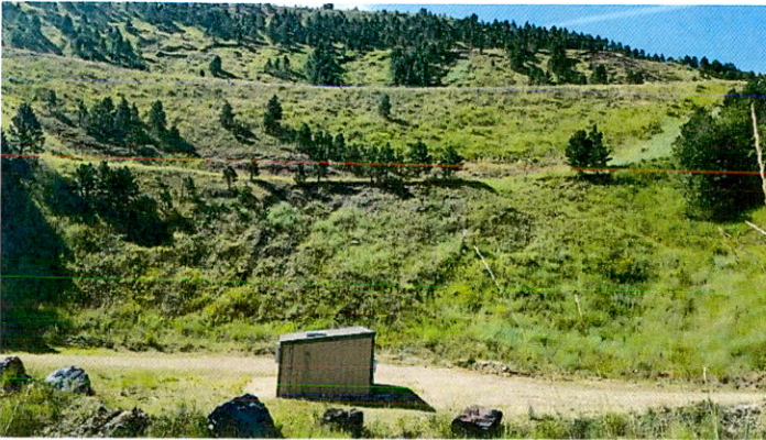
Gayville drainage and pump site
