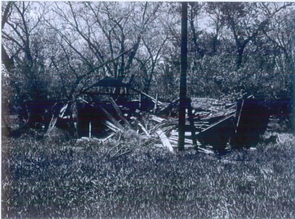
Collapsed sheds facing northwest.
