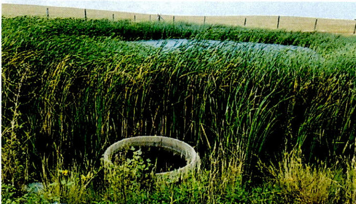
Stilling basin and cooling pond
