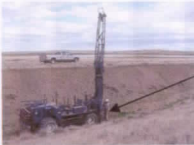
Boring Being Advanced At One Of The Primary Spillway Structure Locations
