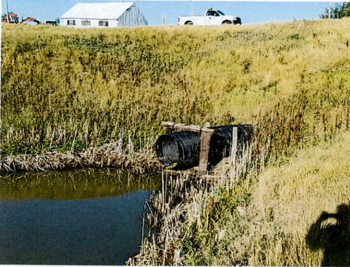
outlet of 48" principal spillway
