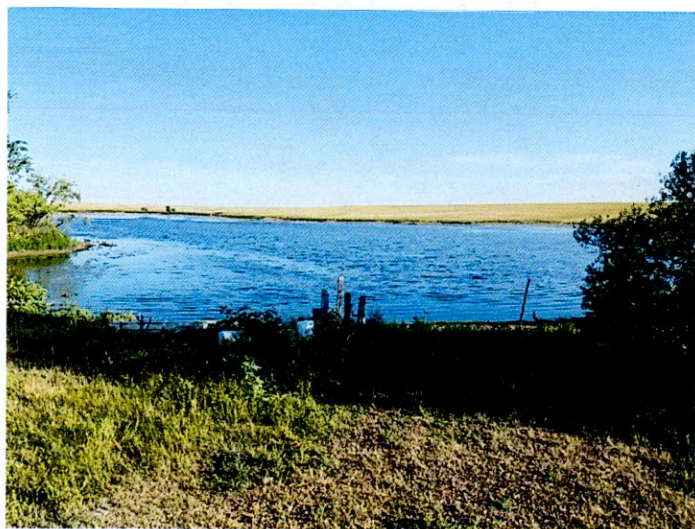
reservoir pool from south end of embankment
