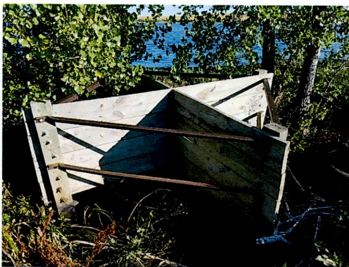
trash rack for principal spillway riser
