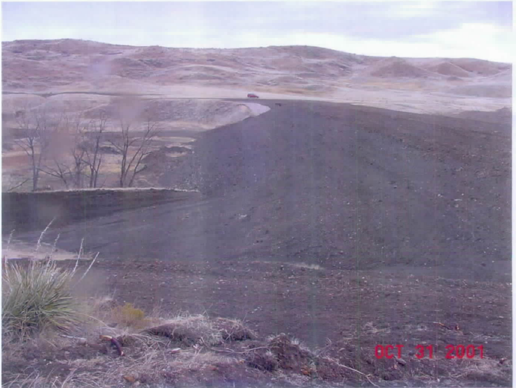
Jim Nelson Dam Upstream slope
