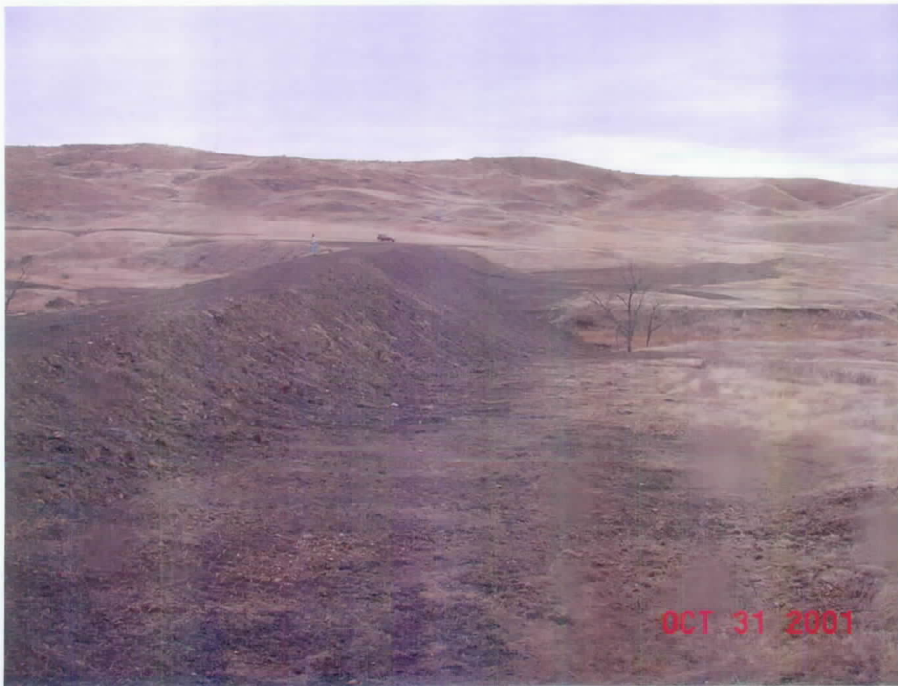
Jim Nelson Dam downstream slope
