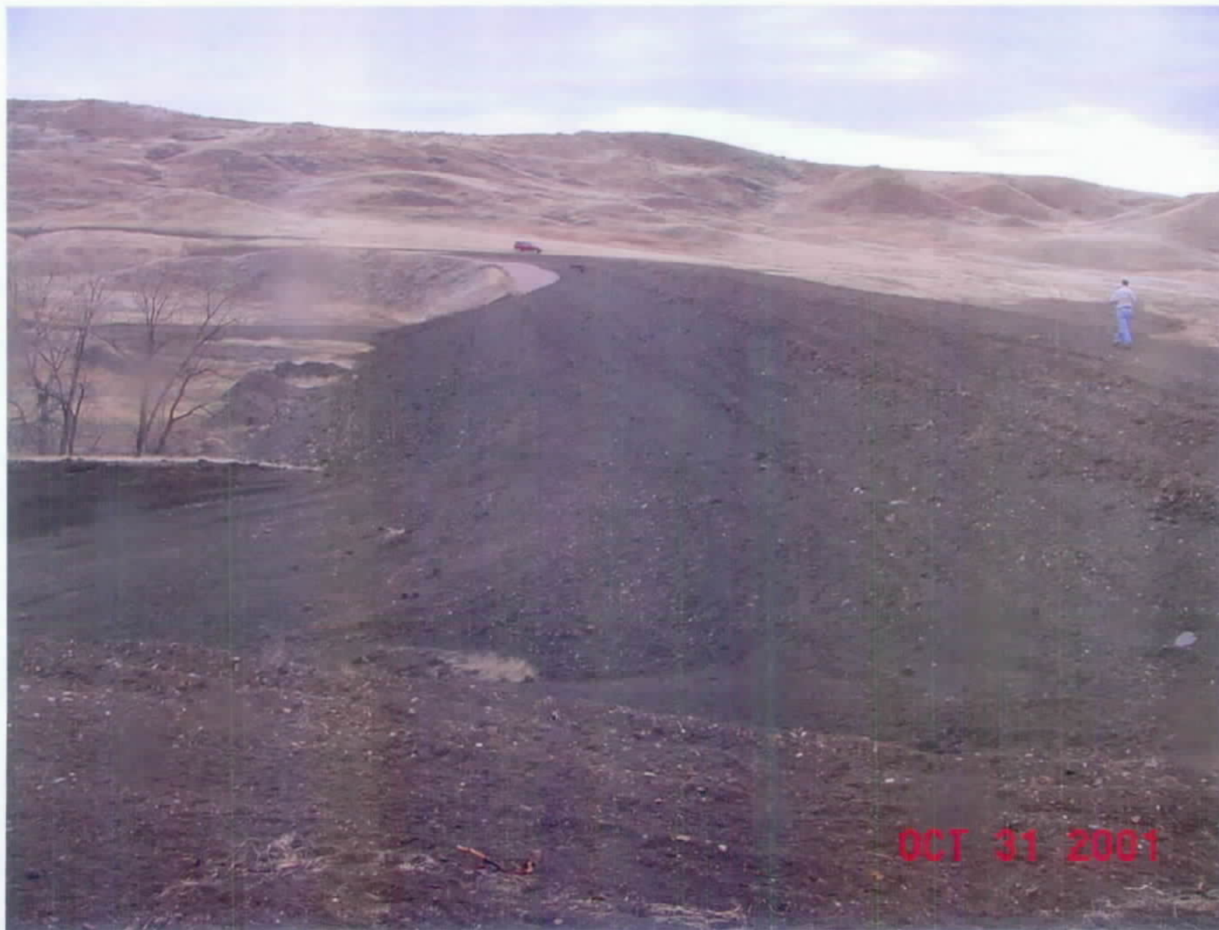
Jim Nelson Dam upstream slope
