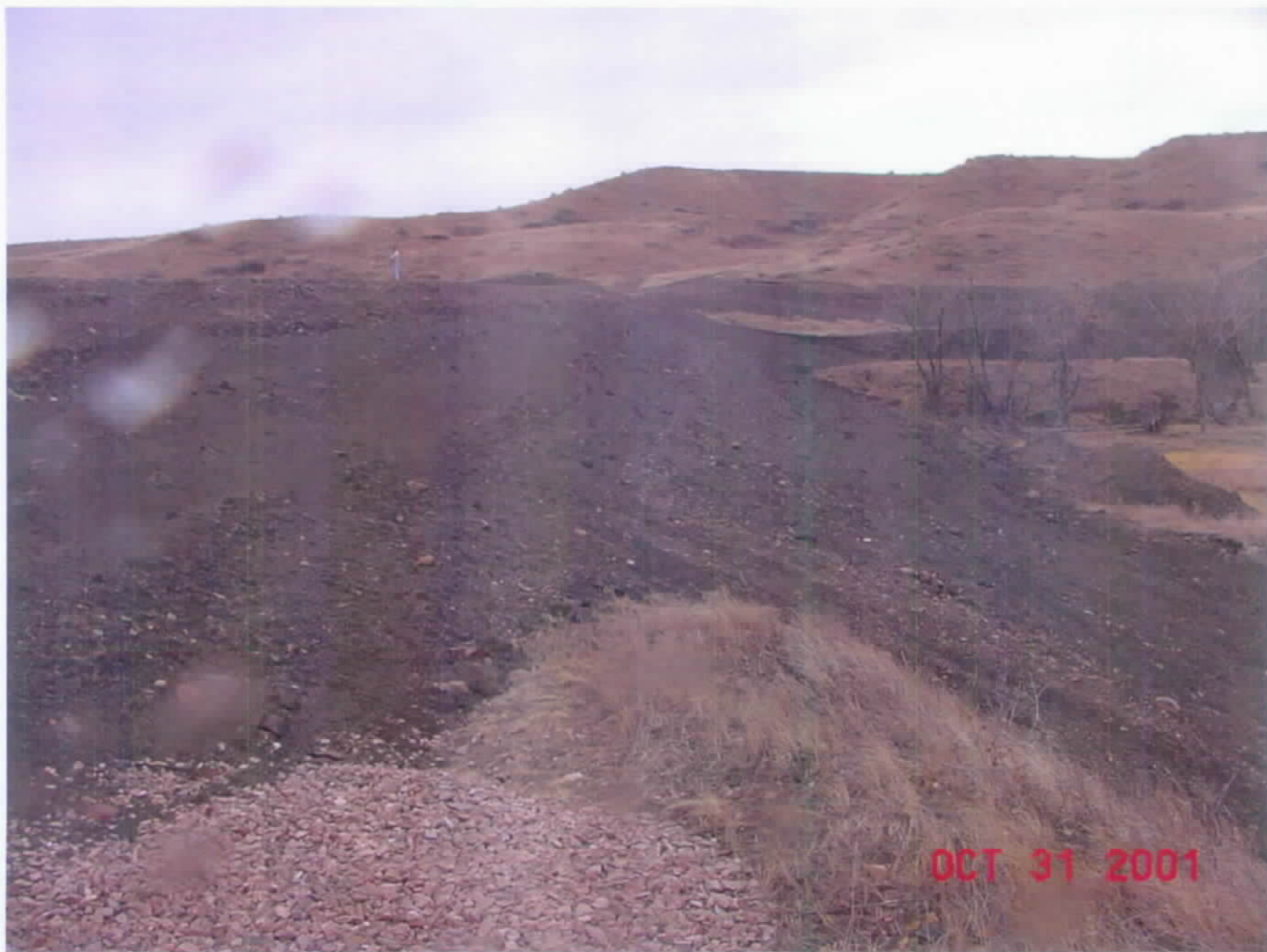
Jim Nelson Dam Upstream slope
