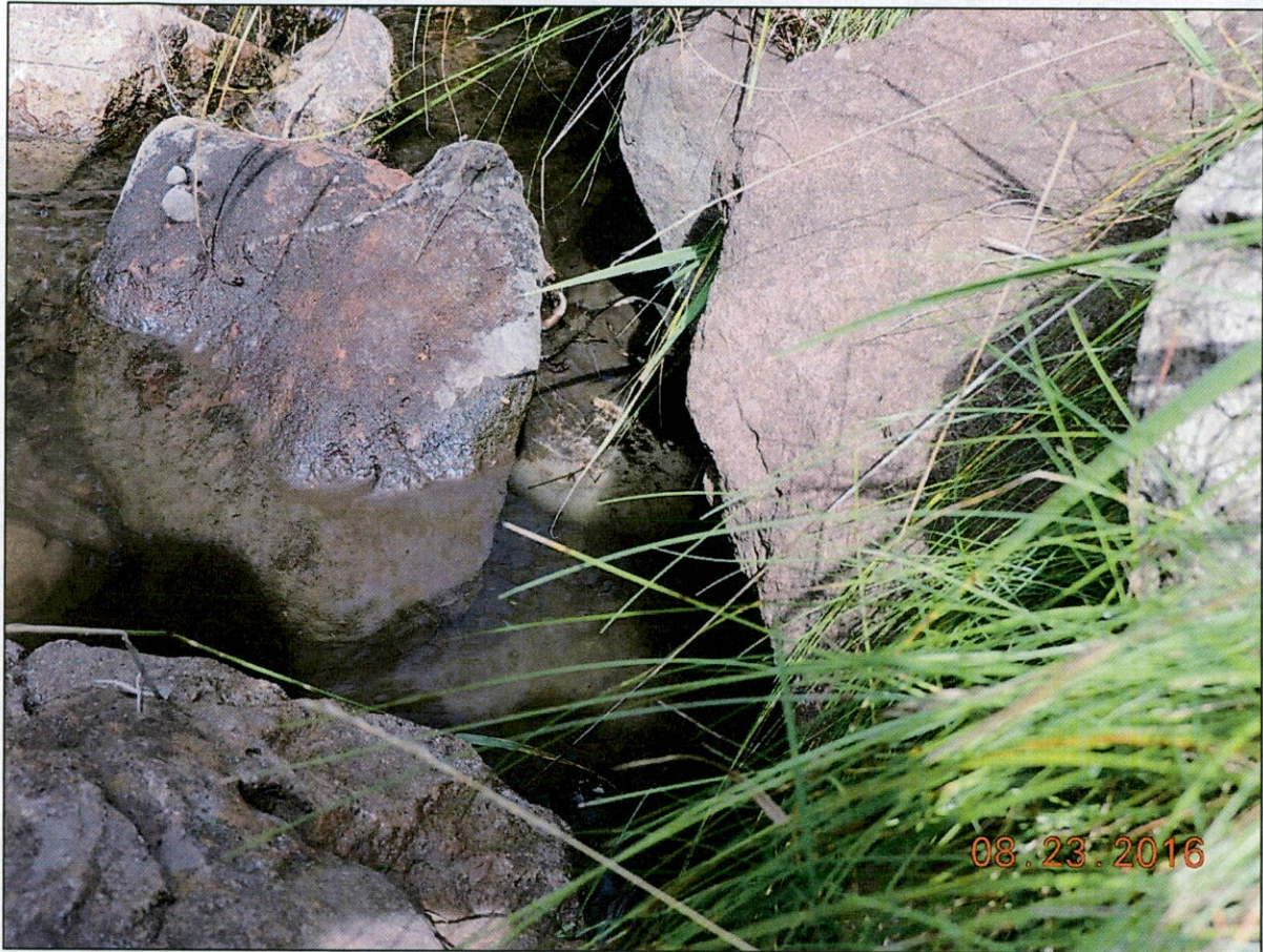
Photo 2 Inlet pipe from Elk Creek.
