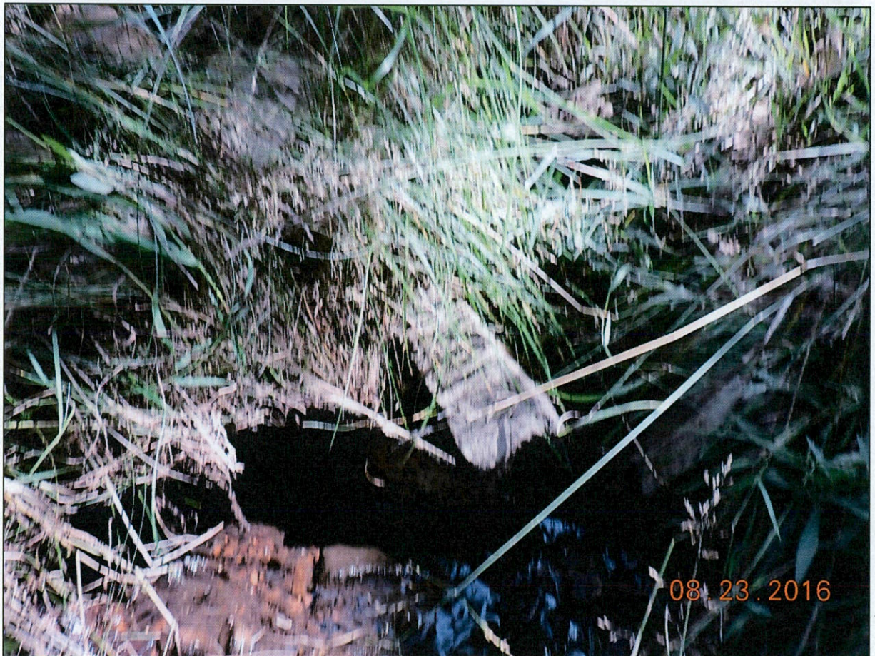
Photo 7 Outlet pipe into Elk Creek.
