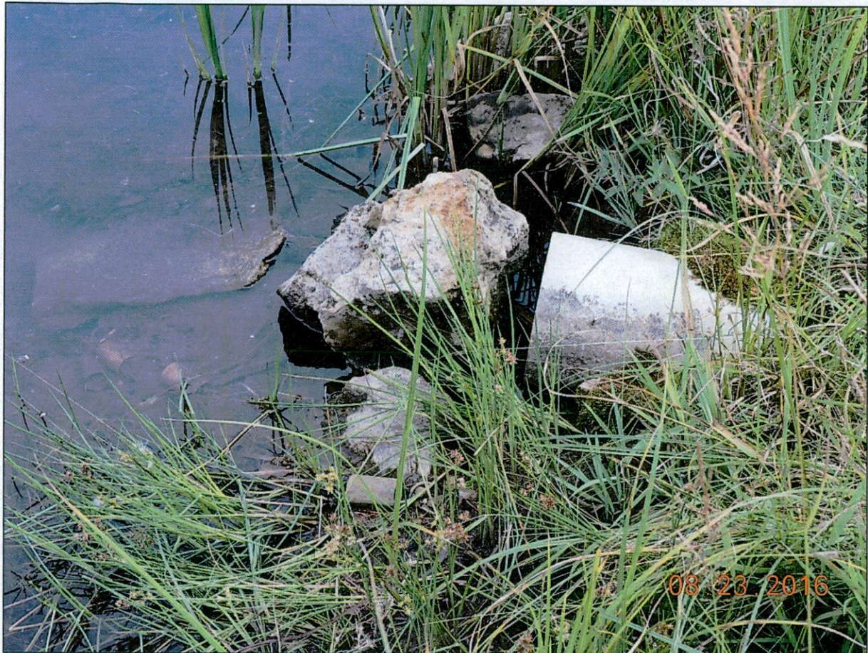
Photo 4 Inlet pipe into the dugout/pond.
