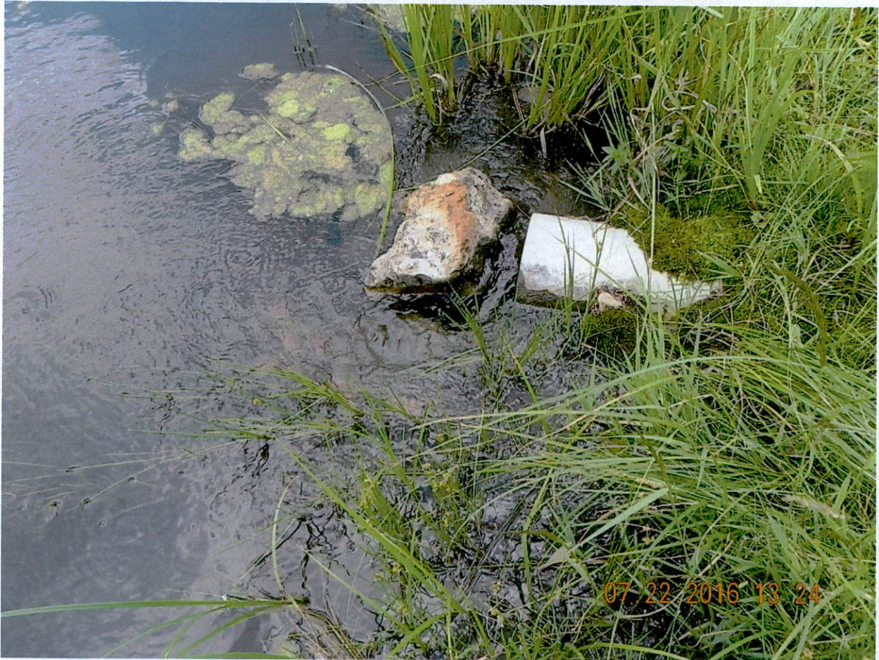
Photo 3 Inlet pipe flow into the pond.
