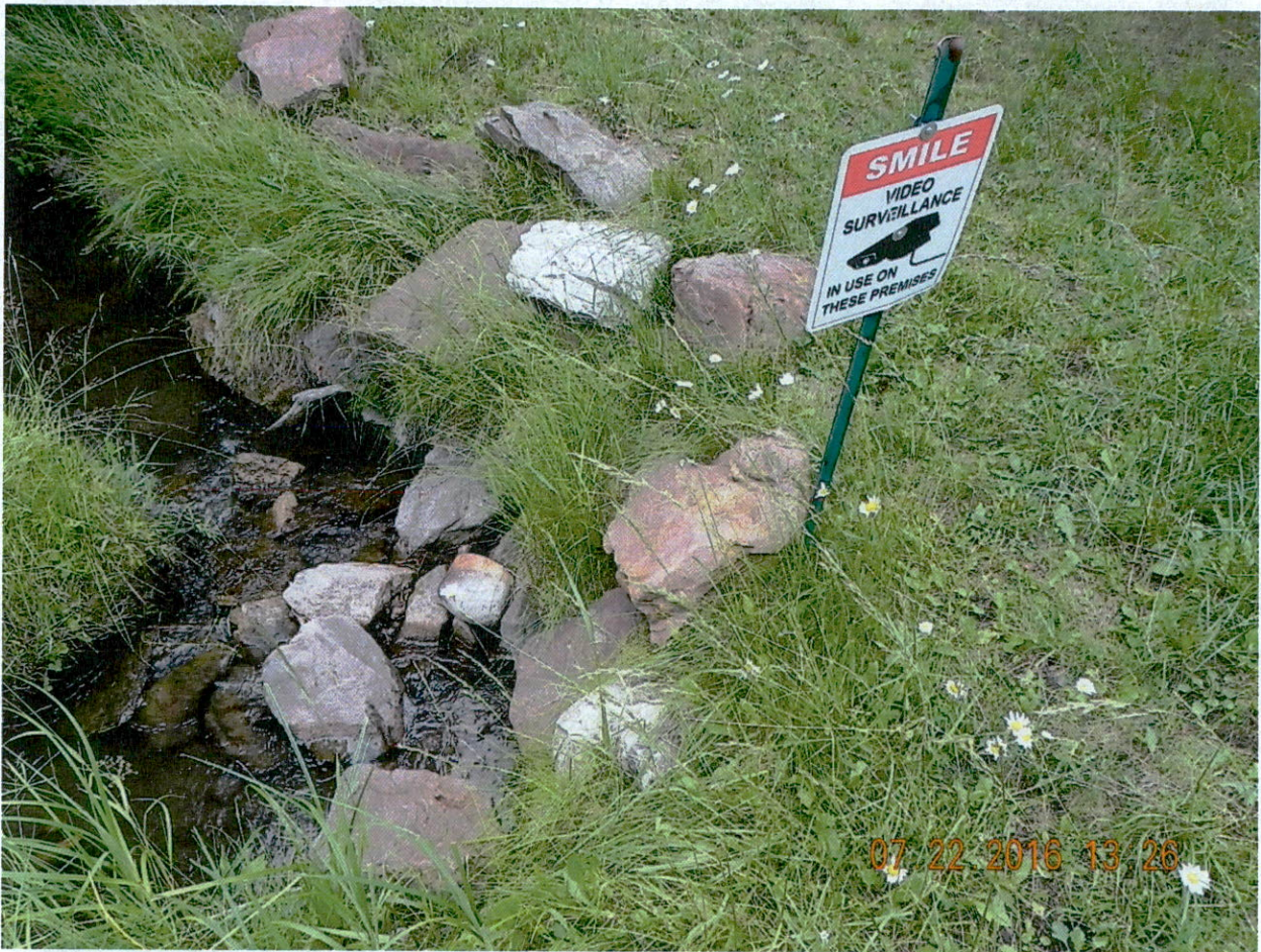
Photo 1 Inlet pipe on Creek Creek.
