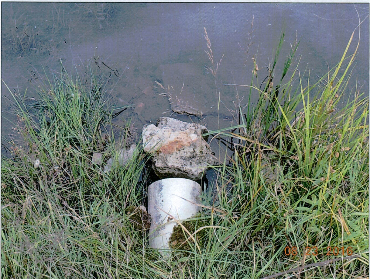
Photo 5 Inlet pipe into the dugout/pond.
