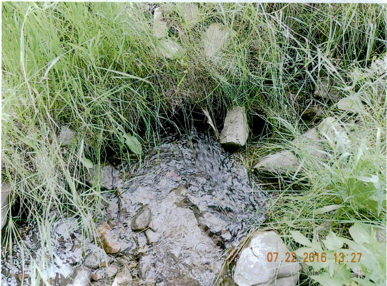
Photo 6 Outlet pipe flow into Elk Creek.
