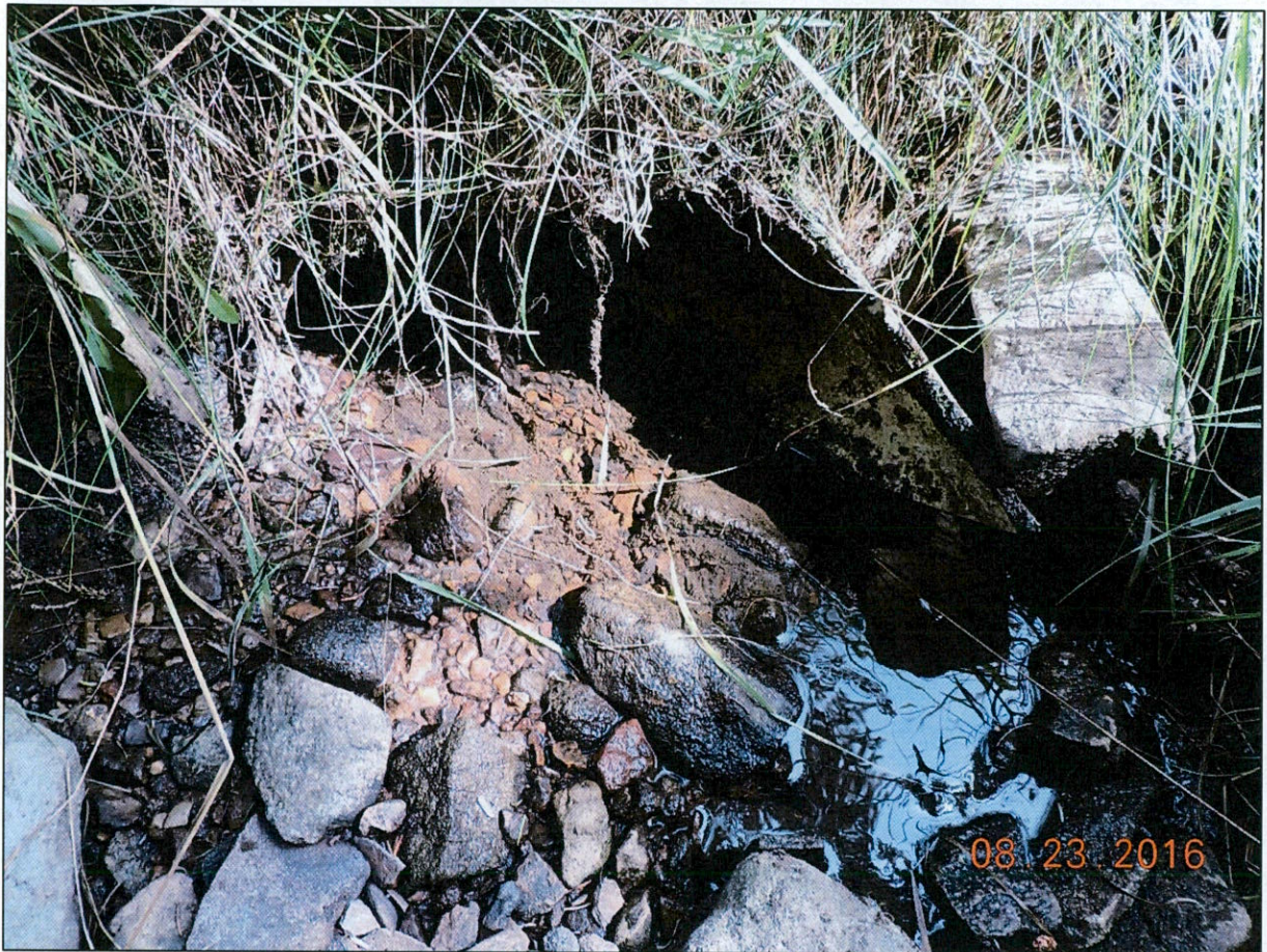
Photo 6 Outlet pipe into Elk Creek.
