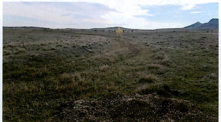
Graded diversion ditch (looking east from diversion dam)
