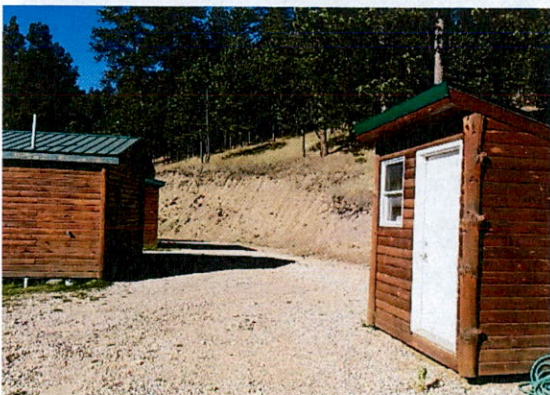
Coles Cabins pump house
