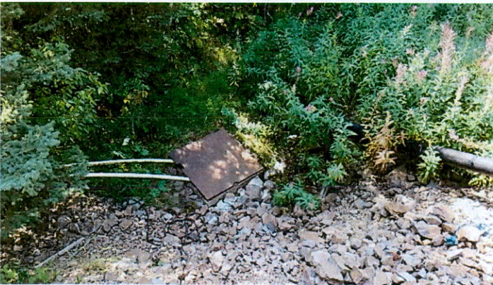
Toe of rock fill embankment in Annie Creek and one of the discharge points for the Ross Valley Denitrification Plant.
