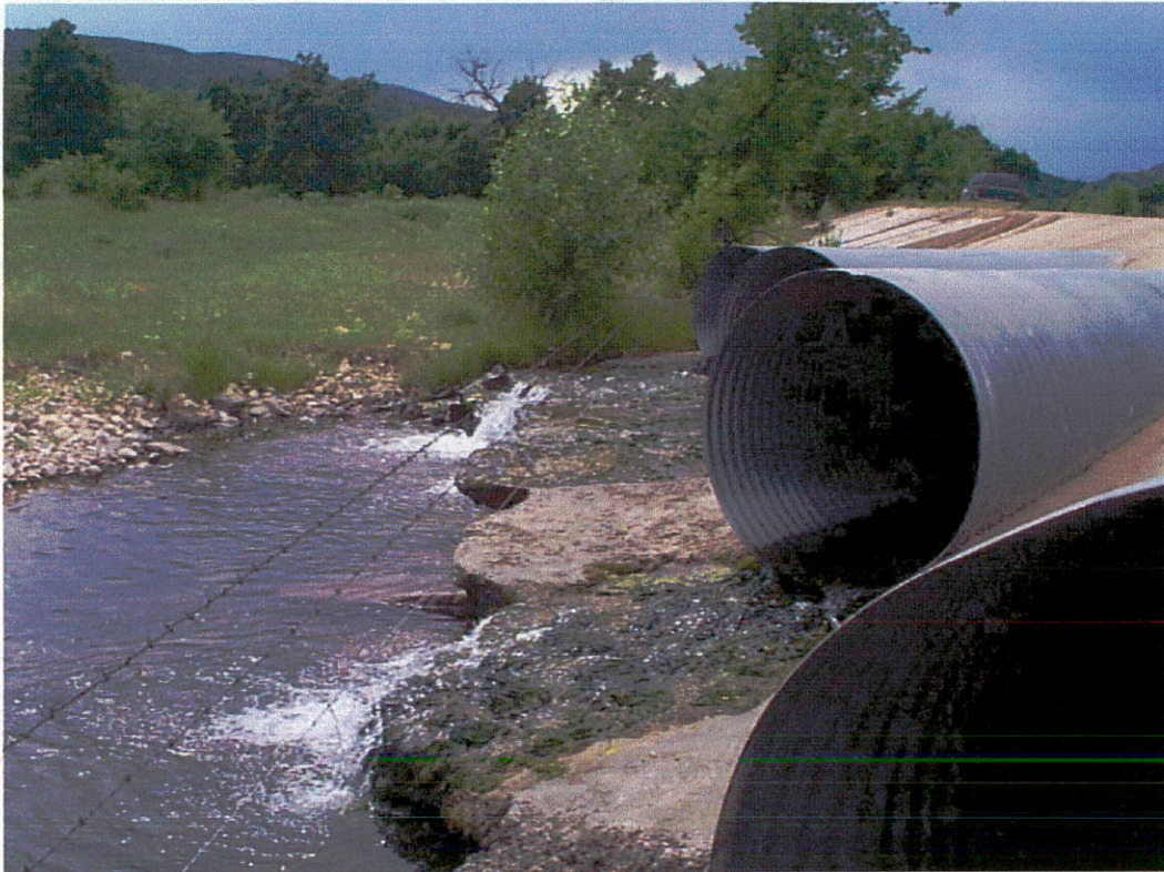
Picture taken looking across 4 culverts located along the Bethlehem Road approximately \frac{3}{4} of a mile west of I-90 bridge (NE \frac{1}{4} NW \frac{1}{4} Sec. 32, T4N, R6E)
