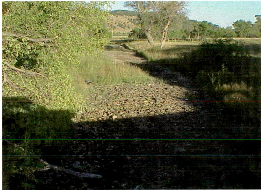
Elk Creek looking downstream on north/south County Road located in the SE \frac{1}{4} SE \frac{1}{4} Section 33, T4N, R6E -- location is approximately 4,800 feet downstream from where Elk Creek crosses I-90
