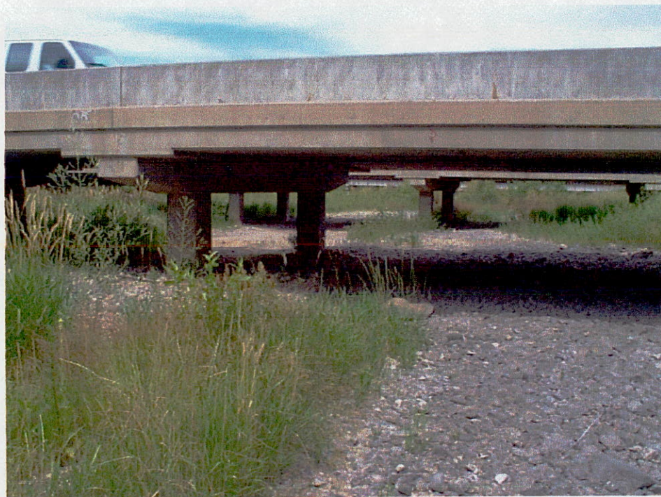
Picture of Elk Creek channel taken looking east (downstream) under the I-90 bridge near the north – south section line between Sections 32 and 33, T4N, R6E
