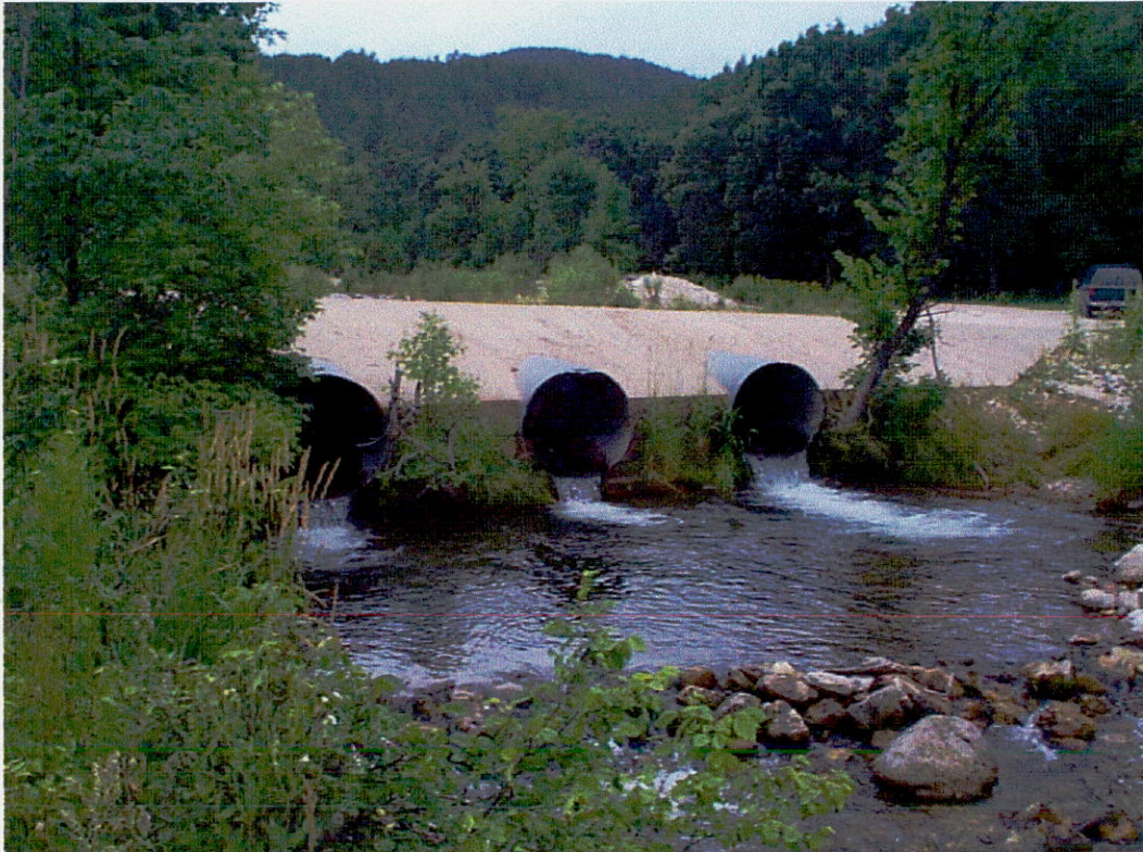
Picture taken at same road crossing as the previous photo showing outfall from the culverts. A few trout were seen in the water at this site.
