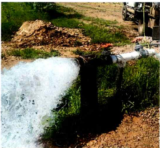
west well @ full flow spring 2016
