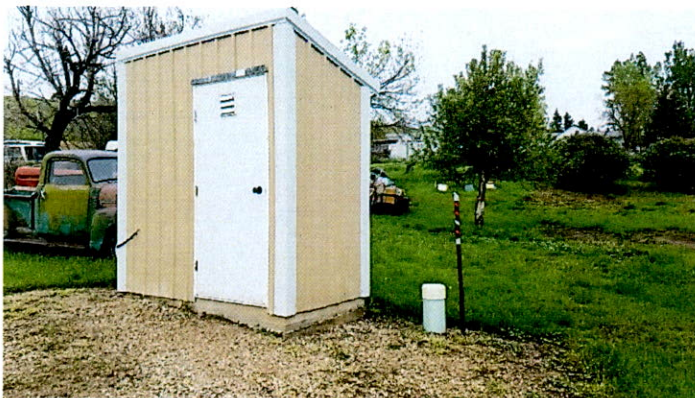
Well and well house over pit
