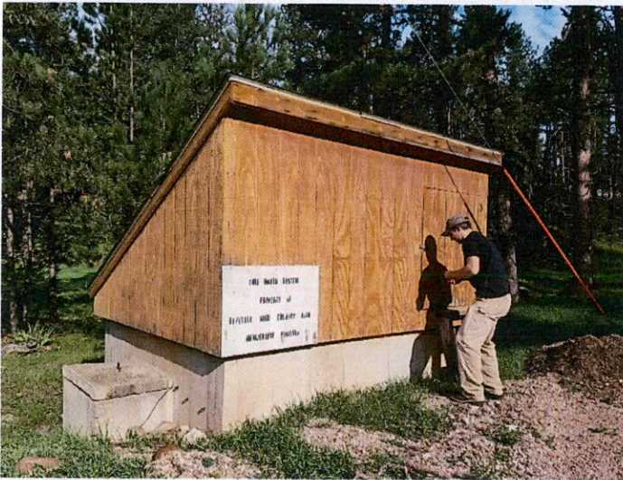
Well house, access for well replacement at left end
